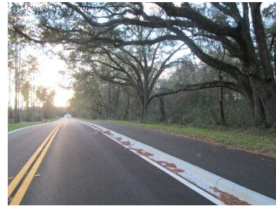
Photo 3: Shared use path along the WEI entrance road connects to U.S. 319
