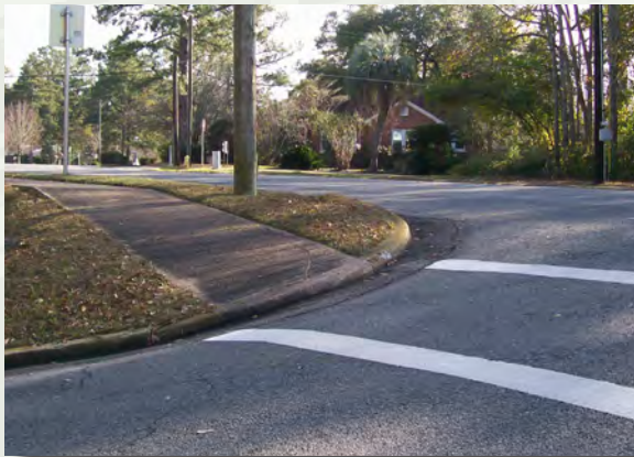
Improper crosswalk segment in Chattahoochee
