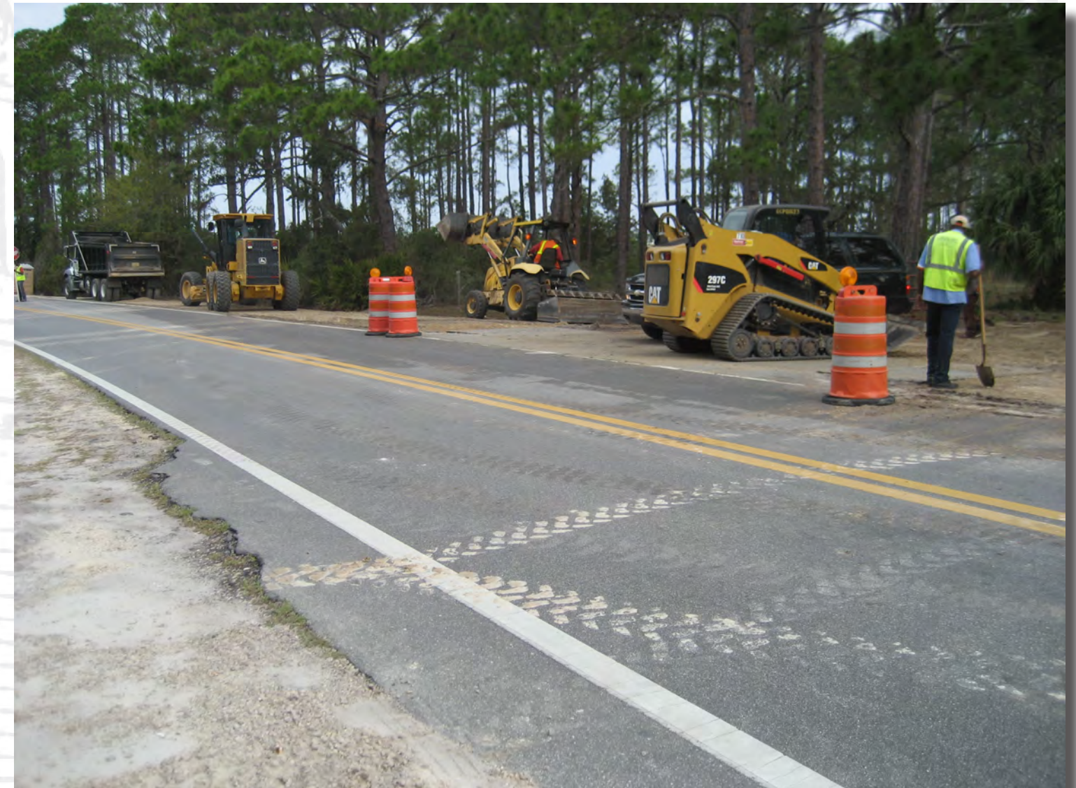
A Shared Use Bicycle Path Under Construction in the Road Right-of-Way
