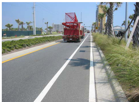
This road in Panama City Beach, FL has 10-foot lanes (which easily accommodate large trucks) adjacent to 5-foot designated bike lanes (4 feet of asphalt, plus gutter pan).
