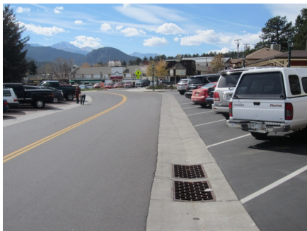
Valley gutters in Estes Park, CO provide a visual separation between angled parking and the travel lanes.
