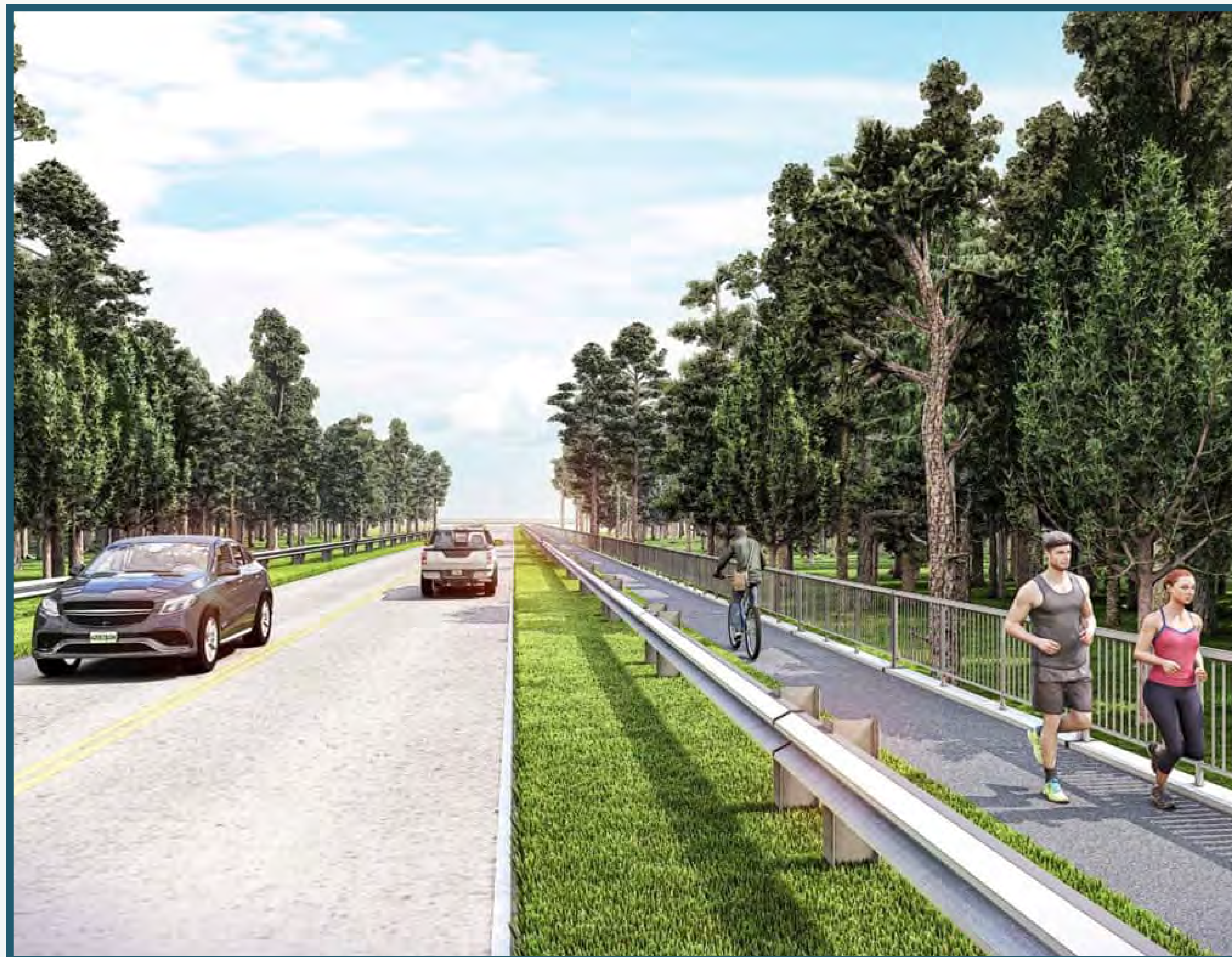
A 10-foot multi-use trail along the east side of Old Bainbridge Road, separated from the roadway by a 7-foot grass shoulder and guardrail.
