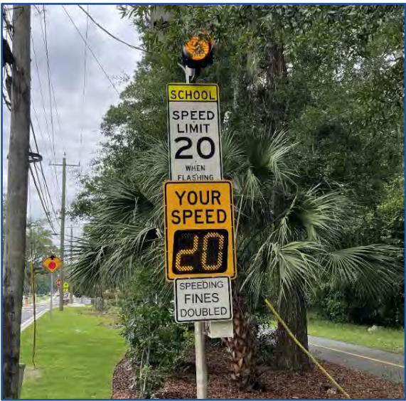
Partially obscured school zone sign flashing beacon on Zillah Street.
