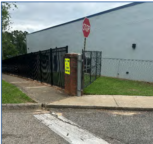
Missing ADA accessible ramp at school exit.
