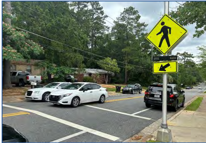
Midblock crosswalk in front of school missing tactile warning strips.
