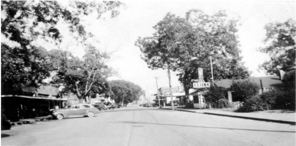
1941 – U.S. 90/Washington Street looking east from Bolivar Street (Source: Florida Archives).
