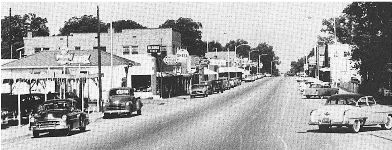
1954 – U.S. 90/Washington Street looking west from Madison Street (Source: Florida Archives).
