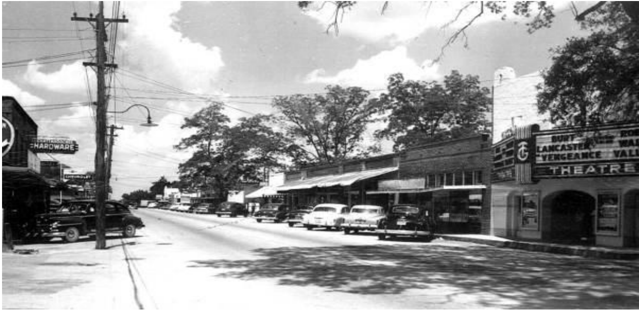
1951 – U.S. 90/Washington Street looking west from Jefferson Street (Source: Florida Archives).
