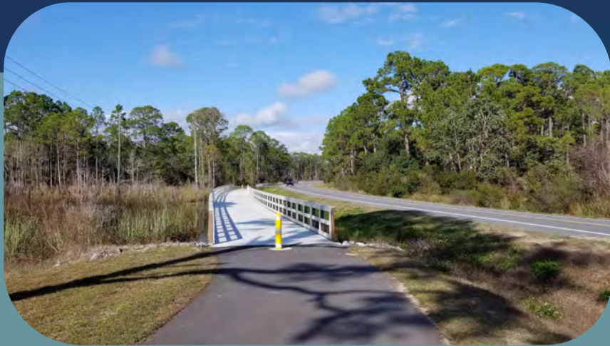
CONSTRUCT NEW BRIDGE
