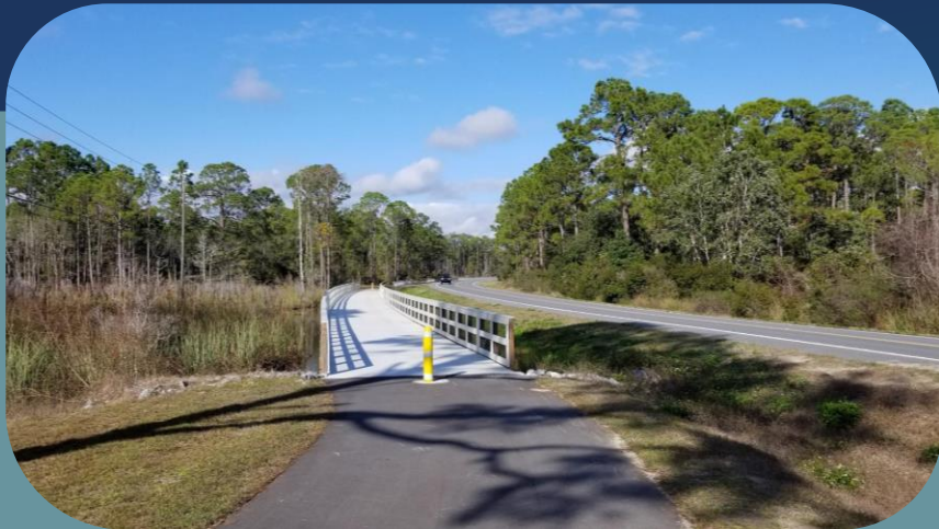
CONSTRUCT NEW BRIDGE
