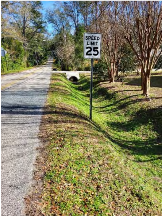
Segments of Waverly Road are flanked by roadside ditches.
