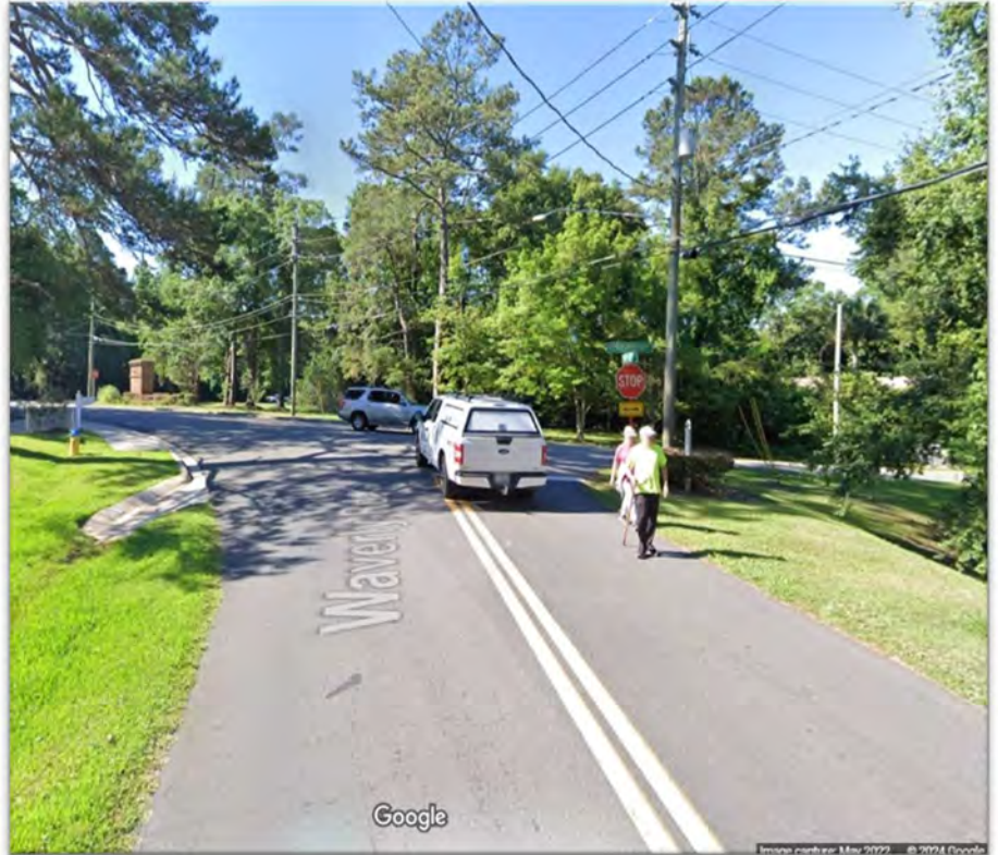
Missing sidewalks along Waverly Road cause pedestrian-vehicle conflicts. Source: Google StreetView, May 2022
