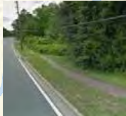
Existing Substandard Sidewalk
