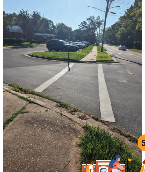
A missing curb ramp on the sidewalk by the student drop-off driveway.
