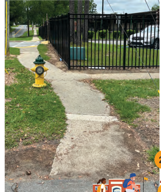
A sidewalk missing a tactile warning strip
