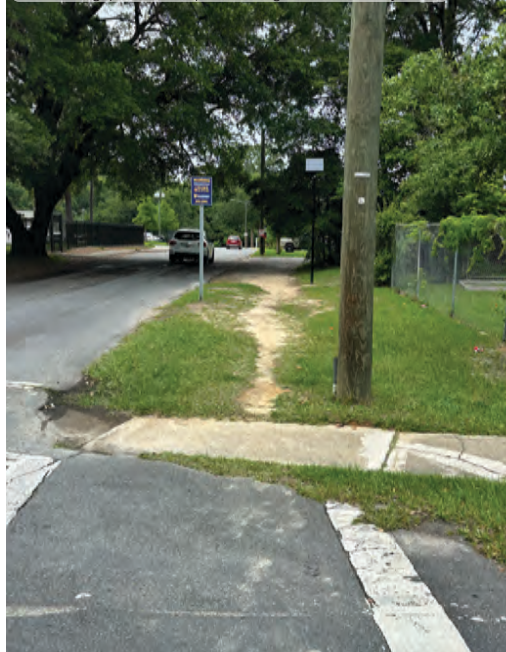
A sidewalk gap with a footpath in the grass on Calloway Street
