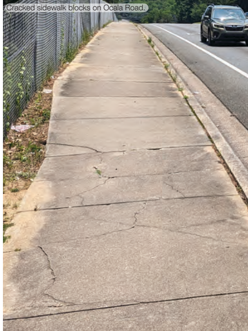
Cracked sidewalk blocks on Ocala Road.
