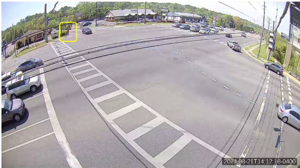
Figure 2: Pedestrian crossing the west approach, poor visibility on the SW corner of the intersection, trees obstructing the view of vehicles and pedestrians (Date 03/21/2024 at 02:12 PM)
