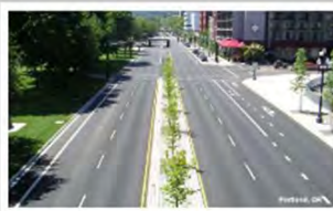
Four-lanes with Multi-Use Path Multi-use path, bike facilities, median
