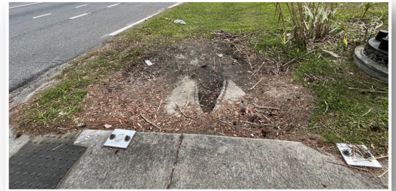
Damaged/Missing Pedestrian Safety Features (No Railing)
