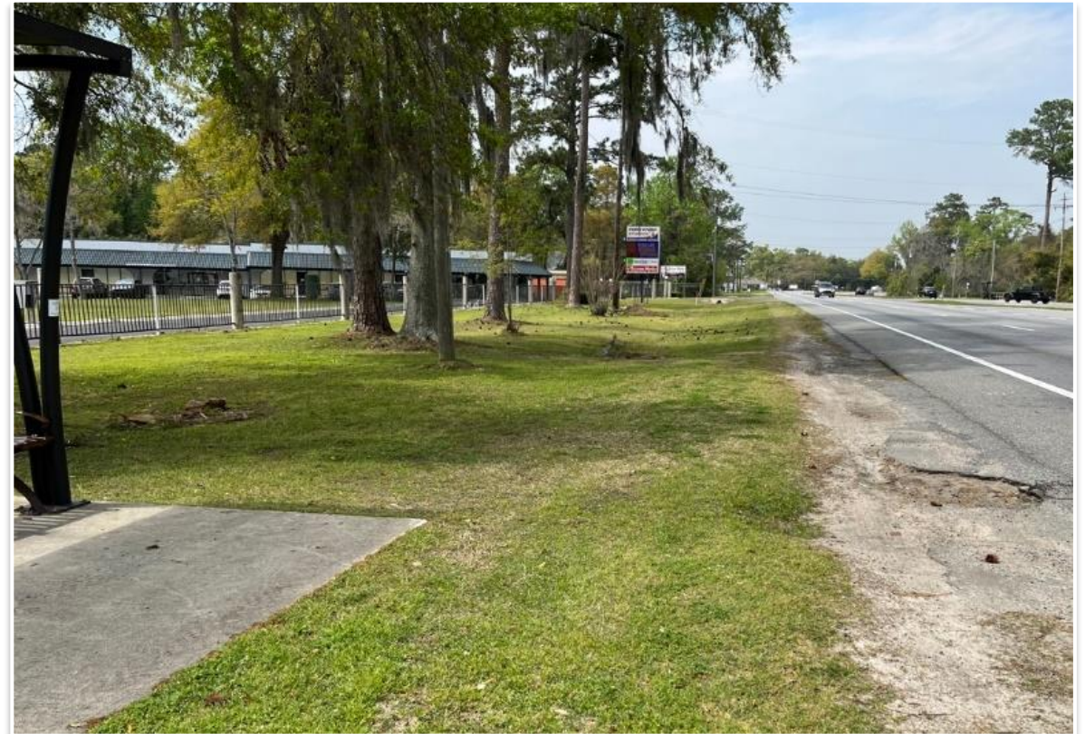
Transit Stop with Limited Pedestrian Access
