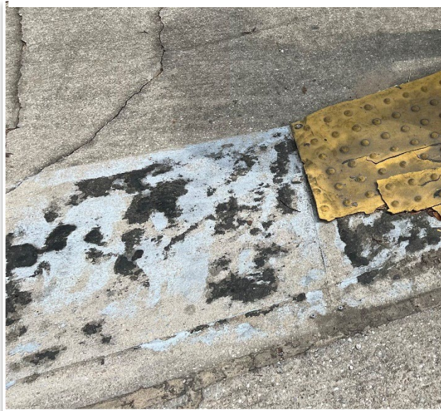
Figure 49: Missing/Damaged Detectable Warning Surface
