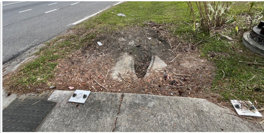
Figure 14: Example of Damaged/Missing Pedestrian Safety Features (no railing)
