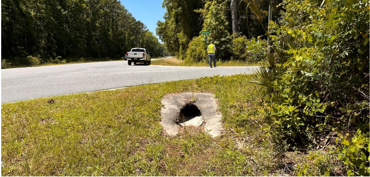
Figure 12: Intersection Drainage Structures (Summerwood Drive)
