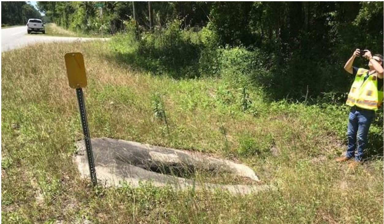
Figure 11: SR 267 – Cross Drains
