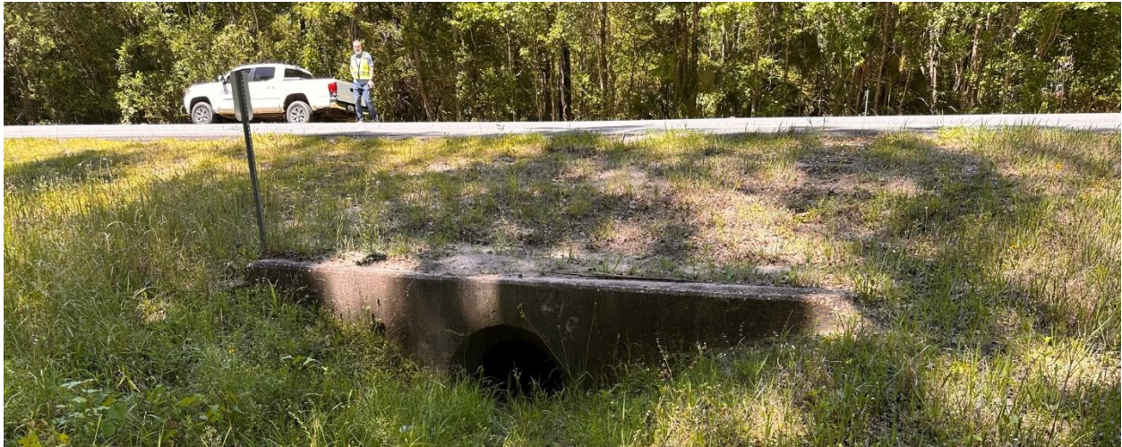
Figure 10: SR 267 – Cross Drain with Headwall
