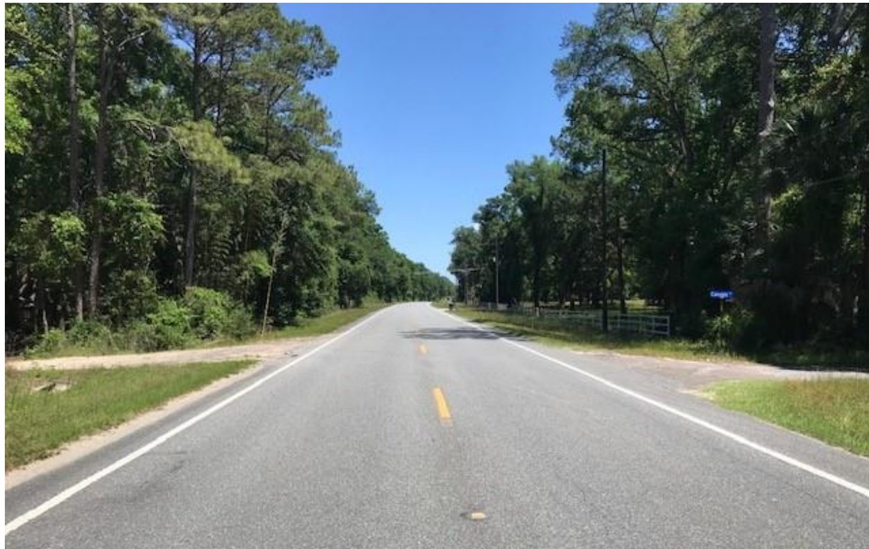
Figure 6: Picture of Existing Typical Section of SR 267
