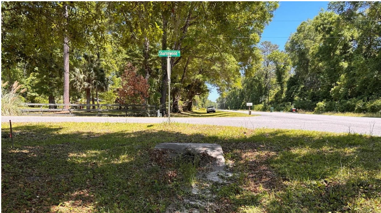
Figure 13: Intersection Drainage Structures (Sharonwood Drive)
