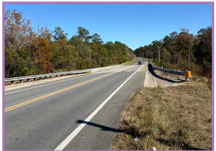
Bridge east of downtown Chattahoochee
