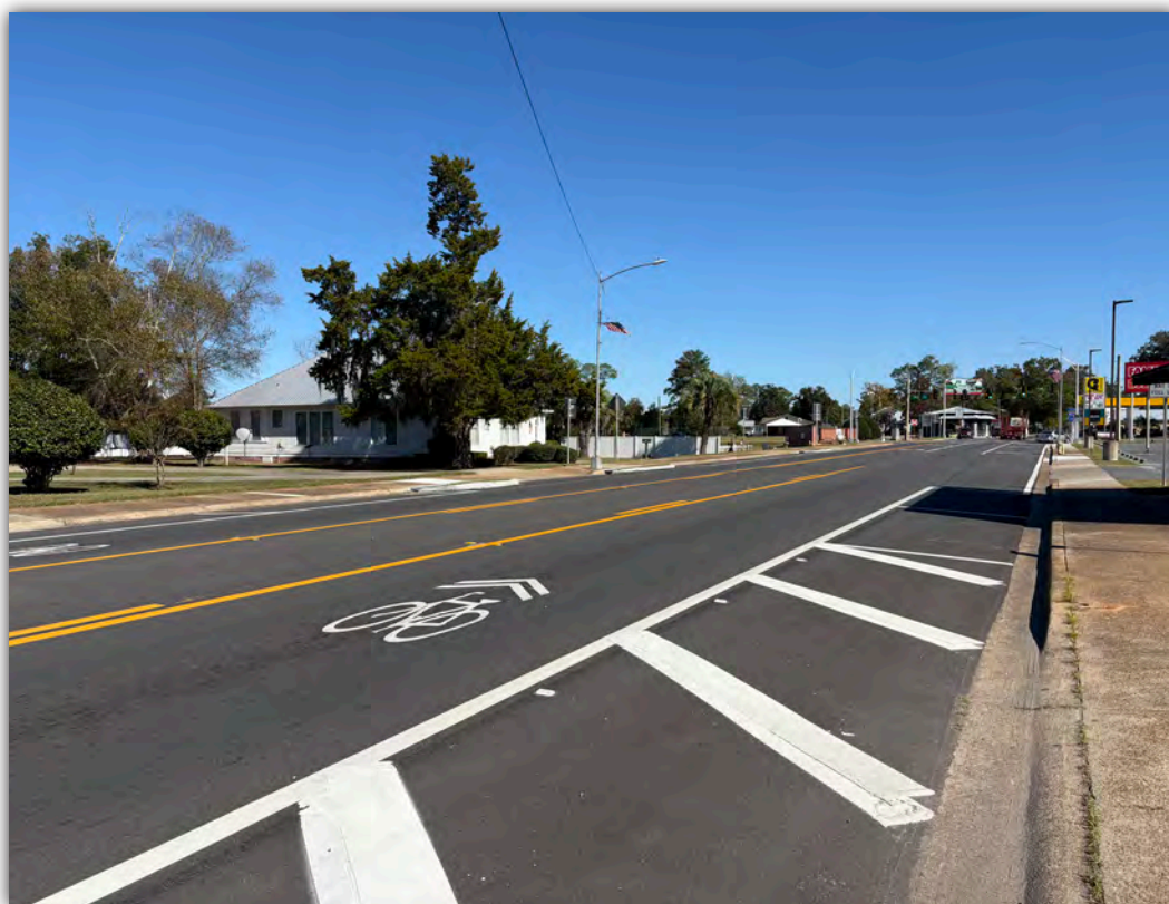
Existing sharrows along US 90 in downtown Chattahoochee
