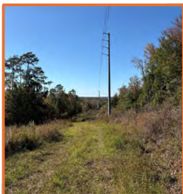
Utility easement south of Chattahoochee
